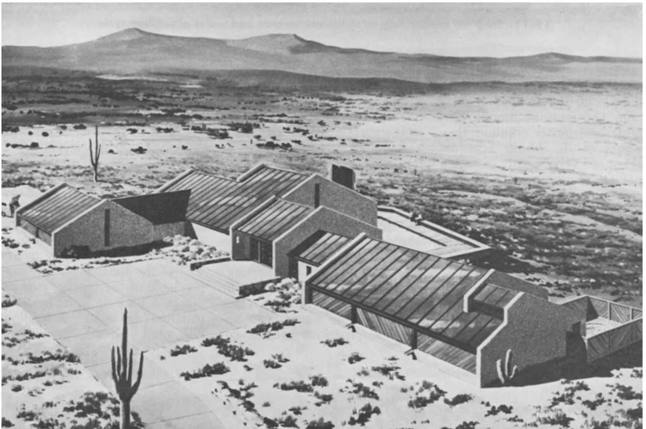
Fig. 17-13 Artist's rendering of a solar house in Tucson, Arizona. The four-bedroom home is cooled by two units fired by solar-heated water. (Arkla)
