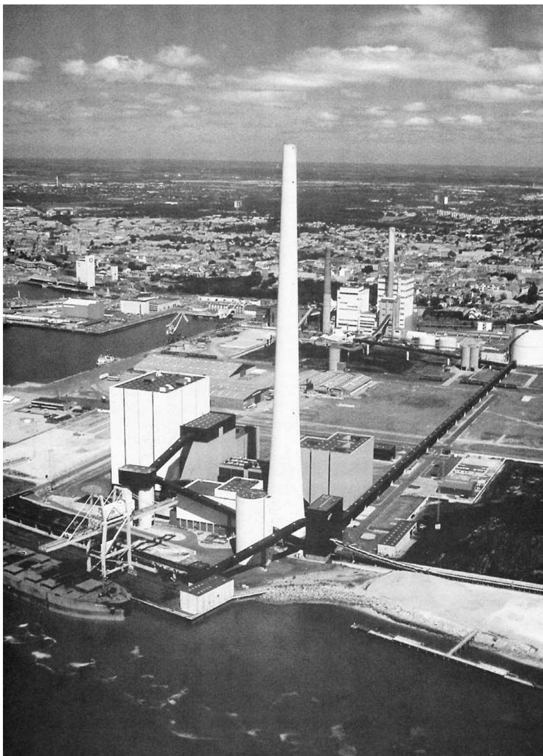
FIGURE 1.2 The Esbjerg, Denmark, power station. (Courtesy Vestkraft 1996.)
