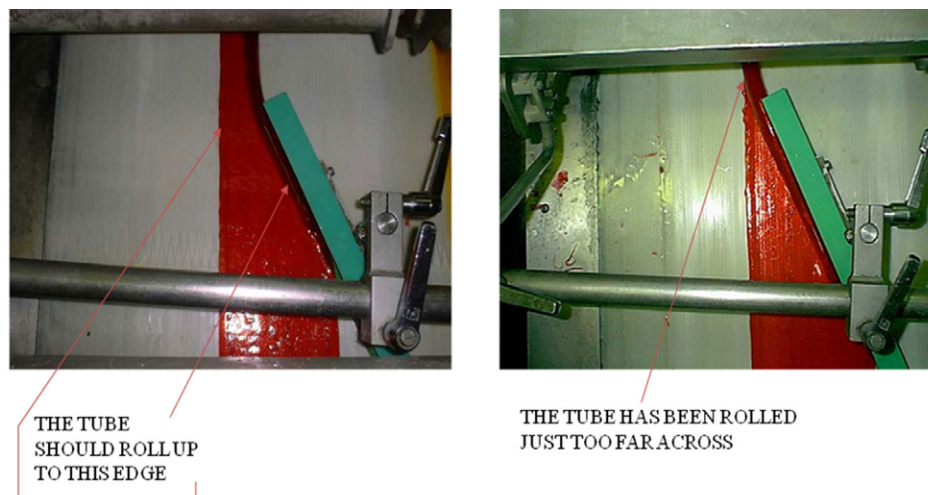
Figure 19.8. Incorrect plough set-up
